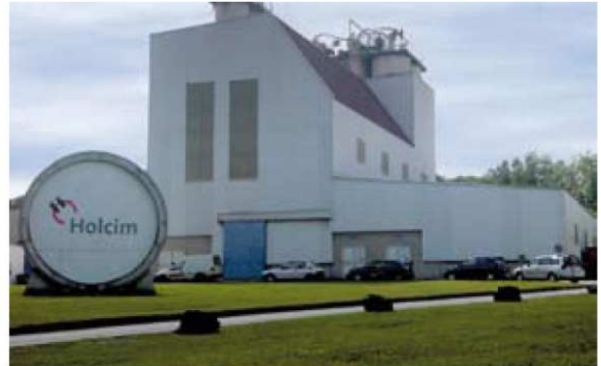
UFB workshop of Lumbres plant.
