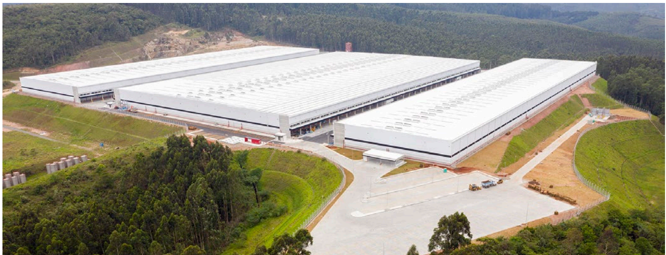
TUF-STRAND SF used in the floor construction of CA35 - Condomínio Anhanguera, Cajamar City, Brazil
