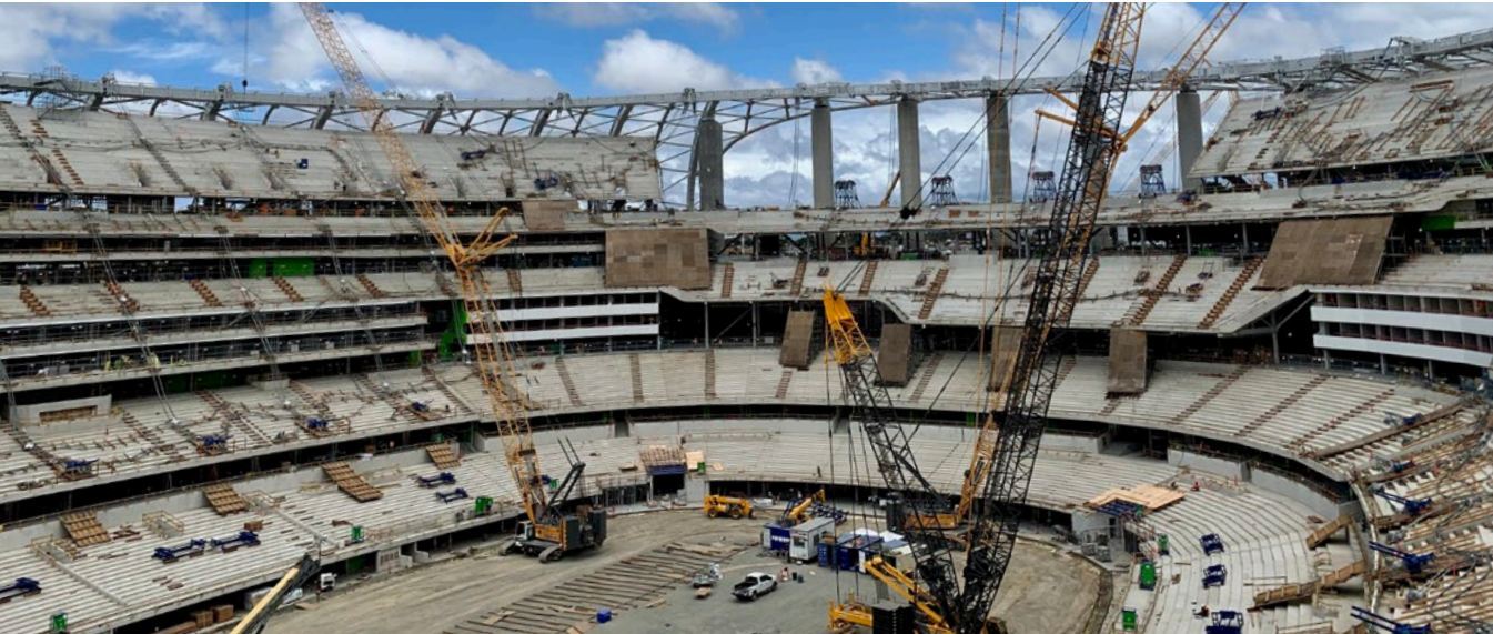
TUF-STRAND SF used in the construction of Sofi Stadium, Inglewood, CA
