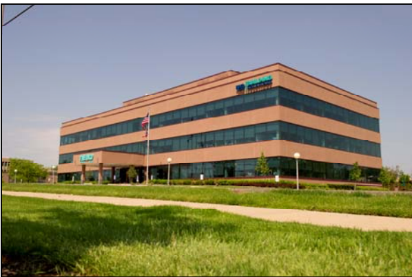
The completed building. Materials from several RPM companies were used, including Dryvit’s Outsulation Plus MD, a decorative and energy-efficient façade.
