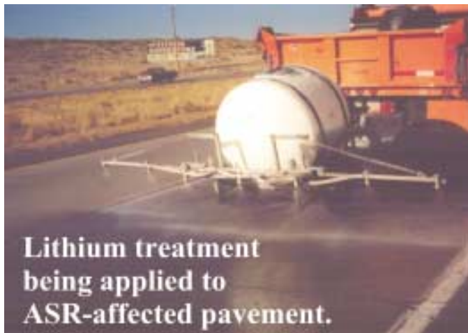
Fig. 4: Lithium-based products may be sprayed on the surface of ASR-affected concrete to further mitigate distress
