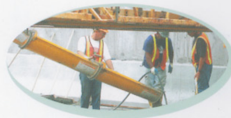
TUF-STRAND SF can be added at the batch plant or on the job site
