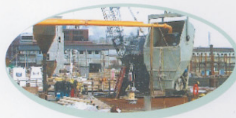
Euclid Chemical admixtures helped maintain pumpability without increasing the water to cement ratio
